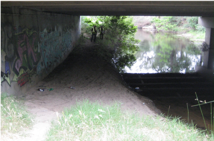
Looking east through Riverside Avenue Bridge
