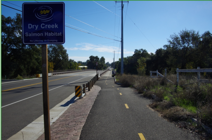
Looking north towards Cook Riolo Road Bridge
